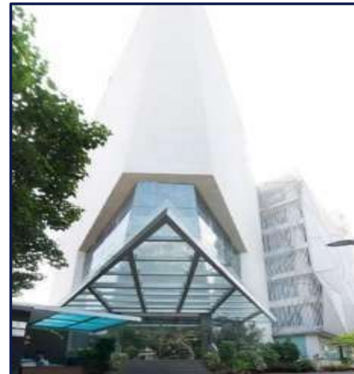
CCIL Bhavan Phase I : Upto 6 th floor
